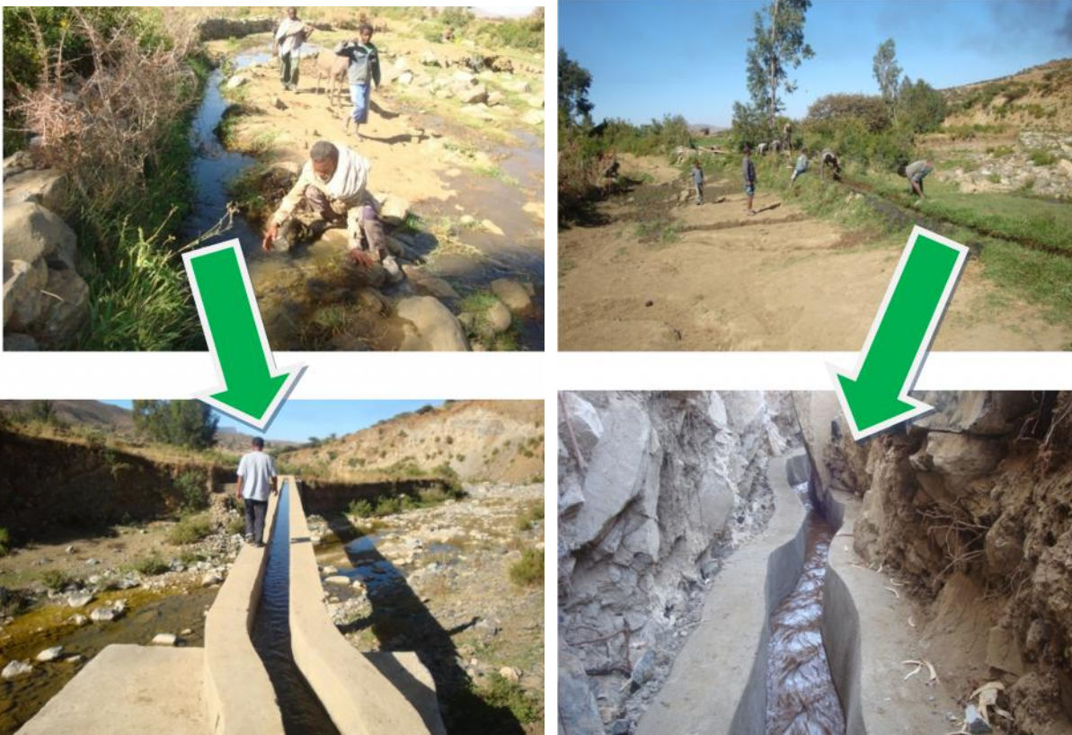
Lined canal for efficient water use and long lasting
